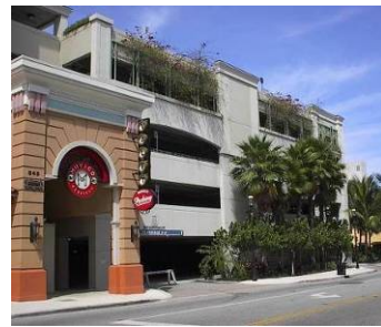
Figure g1. Parking structure with landscaping.
