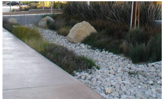
Figure 33. On-site water filtration.
