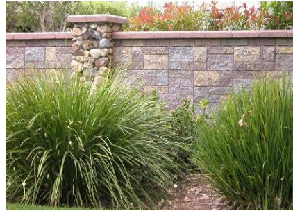
Figure 40. Wall incorporates pilasters and cap.
