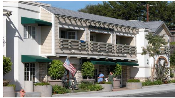
Figure 57. Building elements add visual interest.
