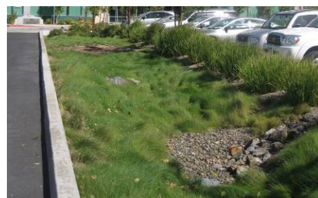
Figure 50. On-site storm water capture.
