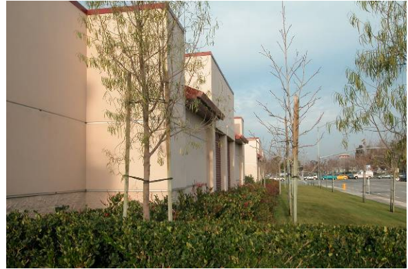
Figure 90. Articulated wall of mini-storage facility.
