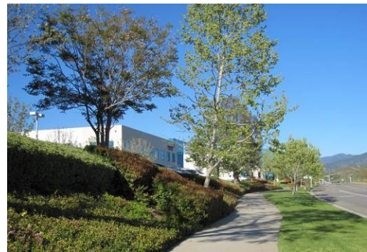
Figure 87. Landscaped berm buffers parking.
