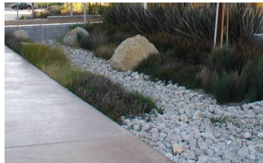
Figure 33. On-site water filtration.
