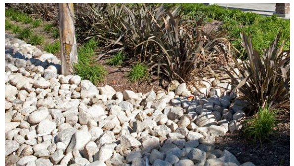
Figure 80. On-site storm water capture system.
