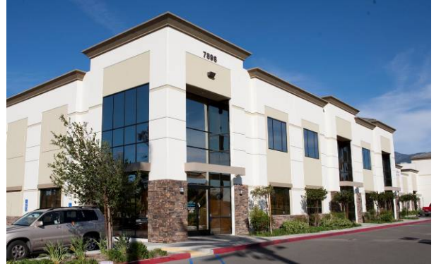
Figure 83. Awnings articulate entries to tenant spaces.
