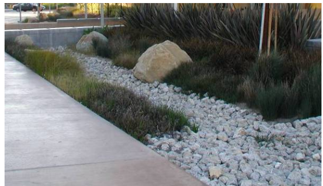
Figure 87. One site water filtration.
