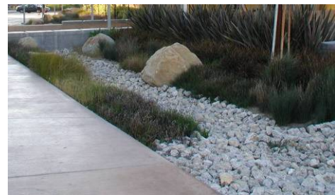
Figure 33. On site water filtration.
