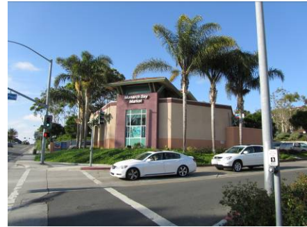
Figure 95. Corner landscaping element.
