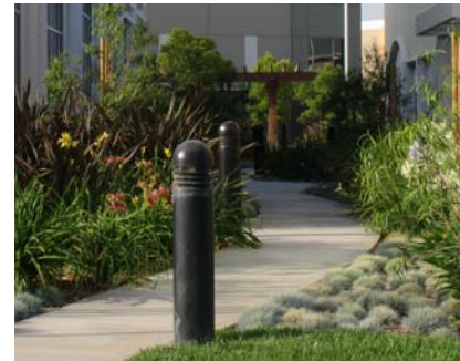
Figure 13. Bollard lighting along pedestrian walkway.
