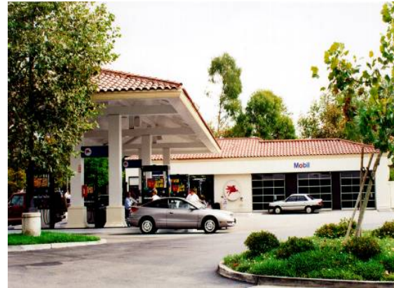
Figure 82. Sloped roof on pump island canopies.
