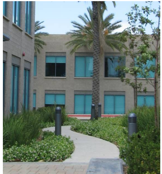
Figure 77. Lighting along pedestrian walkway.
