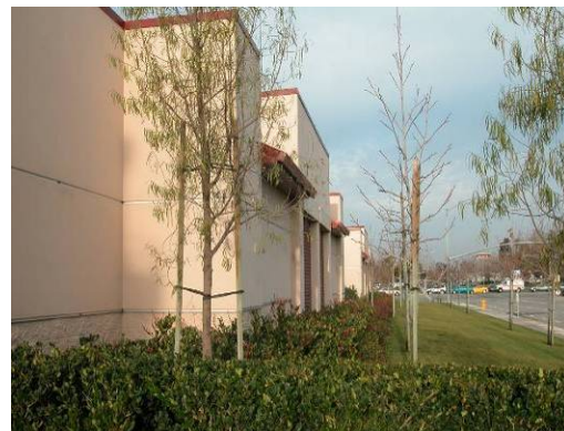
Figure 74. Articulated wall of mini-storage facility.
