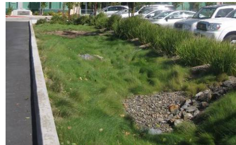
Figure 50. On-site storm water capture.
