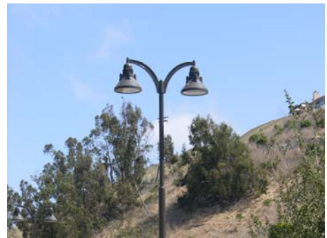
Figure 44. Hooded light fixture directs light downward.
