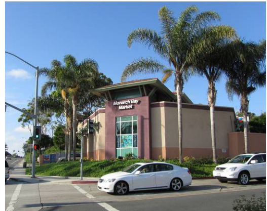
Figure 80. Corner landscaping element.
