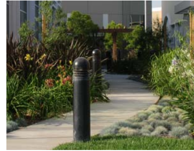
Figure 45. Bollard lighting along pedestrian walkway.
