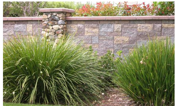
Figure 40. Wall incorporates pilasters and cap.
