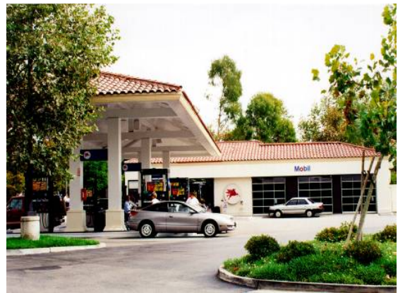
Figure 81. Sloped roof on pump island canopies.
