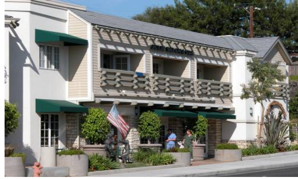
Figure 57. Building elements add visual interest.
