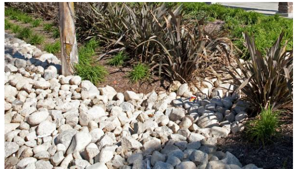
Figure 79. On-site stormwater capture system.
