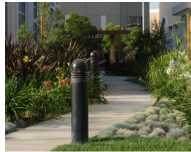
Figure 45. Bollard lighting along pedestrian walkway.
