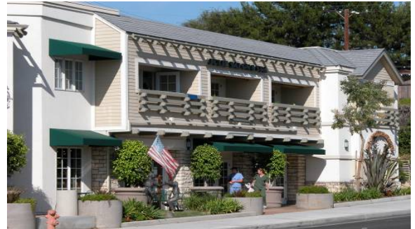
Figure 57. Building elements add visual interest.
