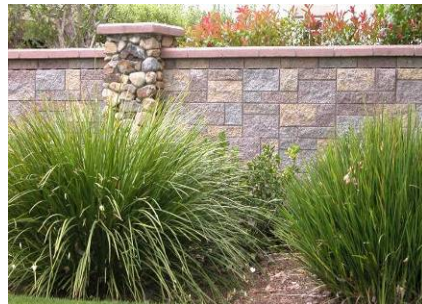
Figure 40. Wall incorporates pilasters and cap.
