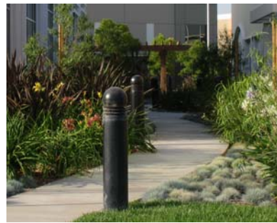
Figure 45. Bollard lighting along pedestrian walkway.
