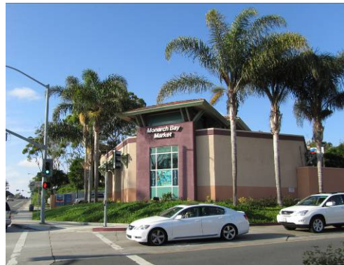
Figure 78. Corner landscaping element.
