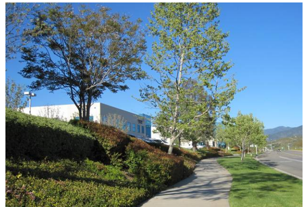
Figure 86. Landscaped berm buffers parking.
