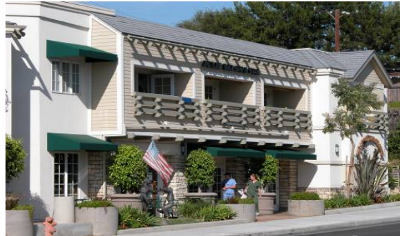
Figure 57. Building elements add visual interest.
