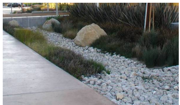
Figure 88. On site water filtration.
