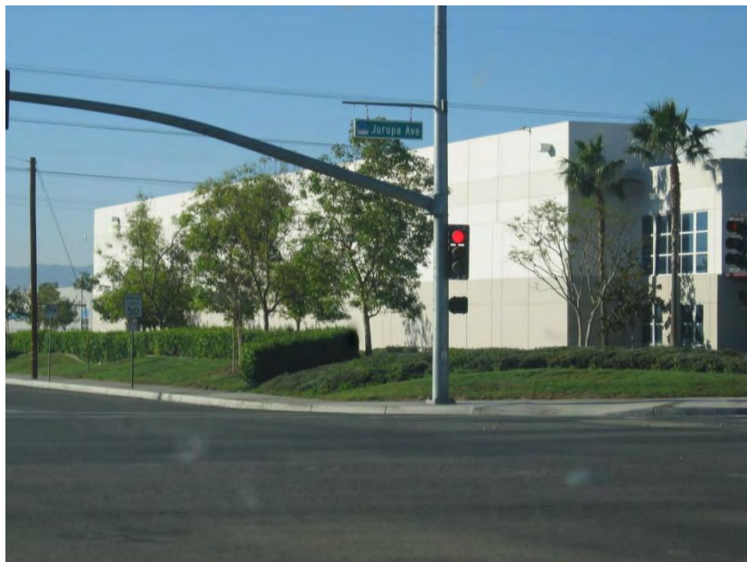
PHOTO 4. Looking at general site conditions of Industrial area along Jurupa Ave.
