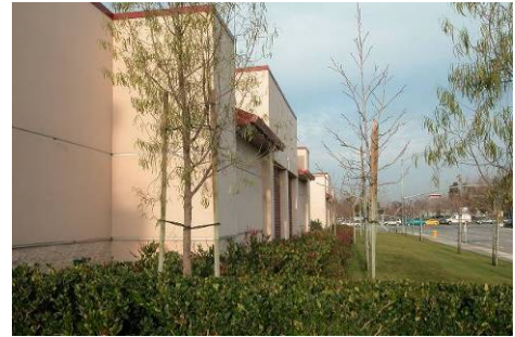
Figure 72. Articulated wall of mini-storage facility.
