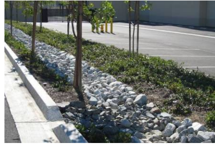
Figure 17. On-site stormwater capture system.
