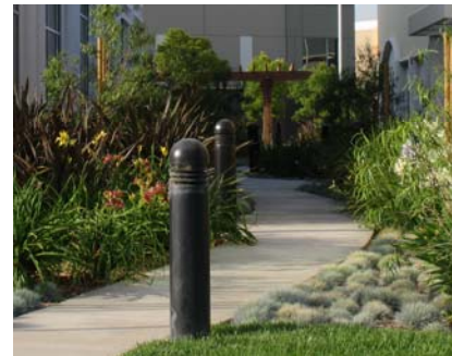
Figure 13. Bollard lighting along pedestrian walkway.
