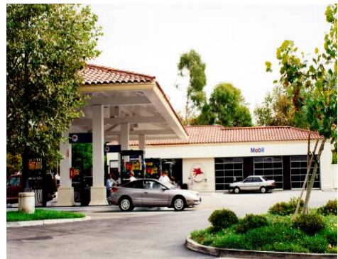
Figure 80. Sloped roof on pump island canopies.
