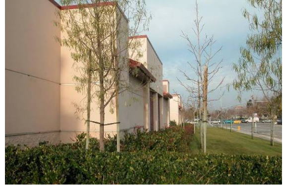
Figure 90. Articulated wall of mini-storage facility.
