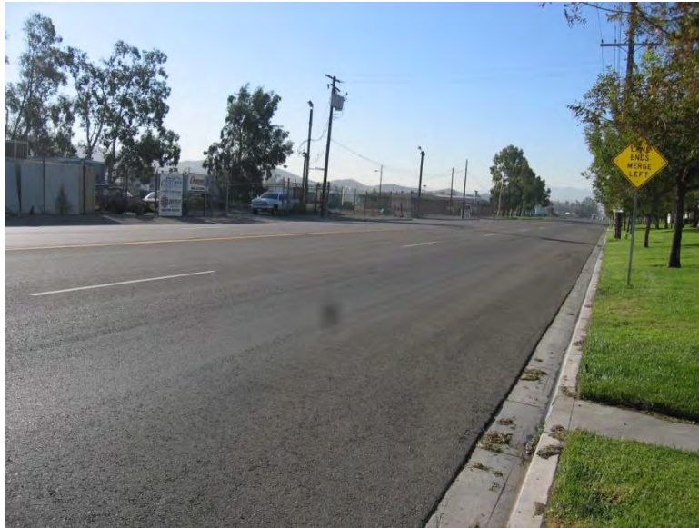
PHOTO 1. Looking southeast along Mulberry Ave. and Slover Ave.
