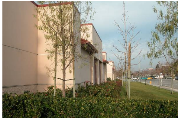
Figure 90. Articulated wall of mini-storage facility.
