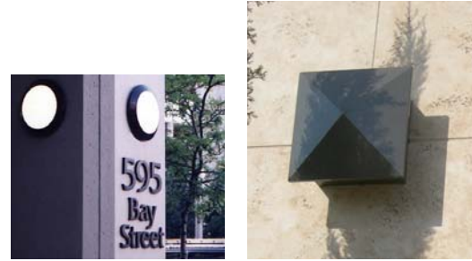
Figure 47. Decorative light fixtures.
