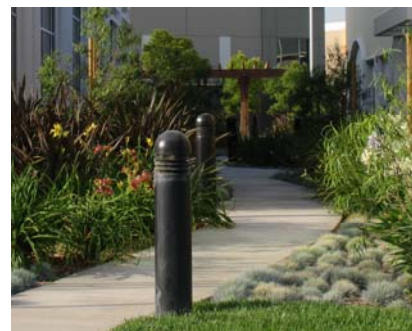
Figure 13. Bollard lighting along pedestrian walkway.
