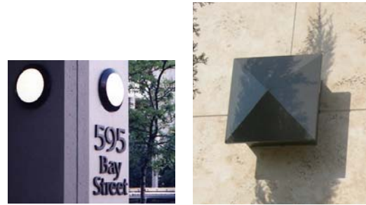
Figure 47. Decorative light fixtures.
