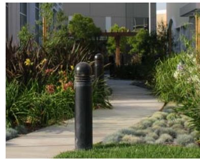
Figure 45. Bollard lighting along pedestrian walkway.
