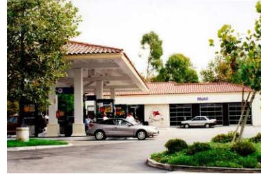
Figure 97. Sloped roof on pump island canopies.
