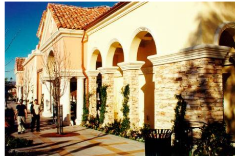
Figure 85. Articulation along wall plane.
