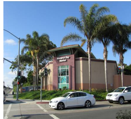
Figure 79. Corner landscaping element.
