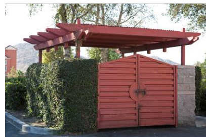
Figure 11. Trash enclosures with architectural screening elements.
