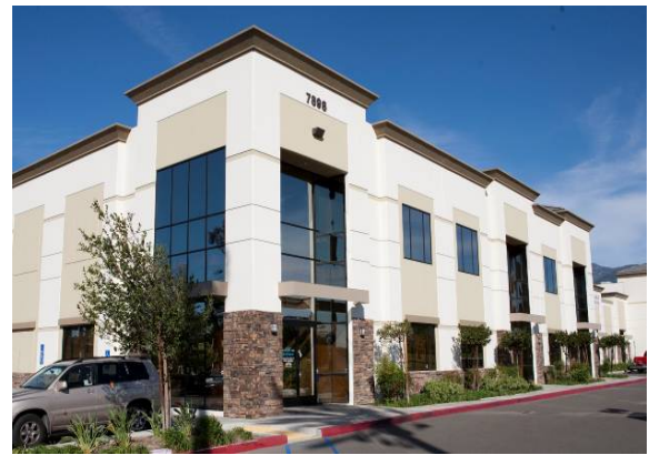
Figure 83. Awnings articulate entries to tenant spaces.
