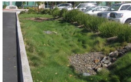
Figure 50. On-site storm water capture.
