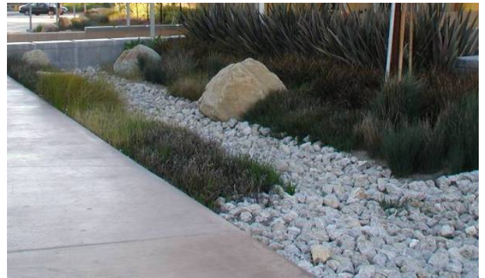
Figure 87. On-site water filtration.
