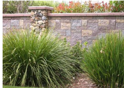
Figure 40. Wall incorporates pilasters and cap.
