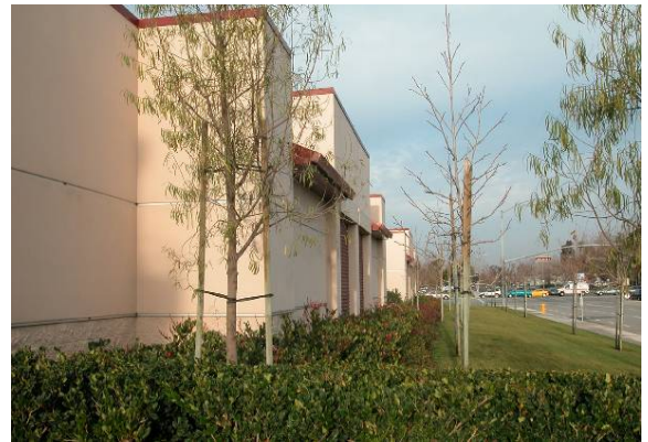
Figure 74. Articulated wall of mini-storage facility.
