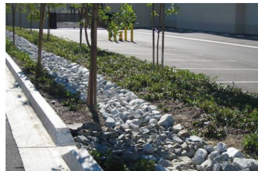
Figure 17. On-site storm water capture system.
