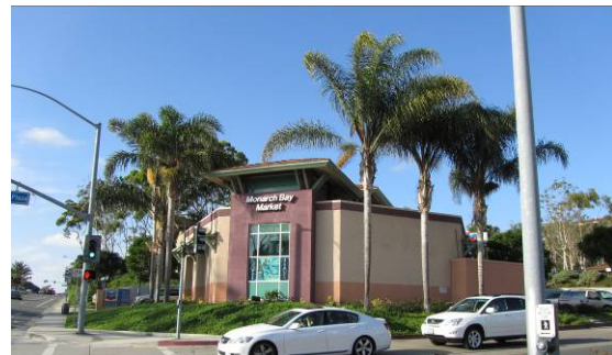
Figure 96. Corner landscaping element.
