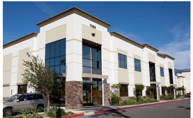
Figure 84. Awnings articulate entries to tenant spaces.
