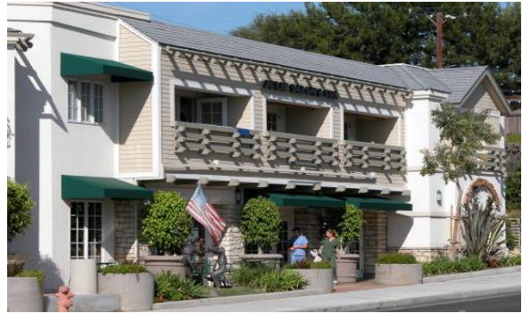
Figure 57. Building elements add visual interest.
