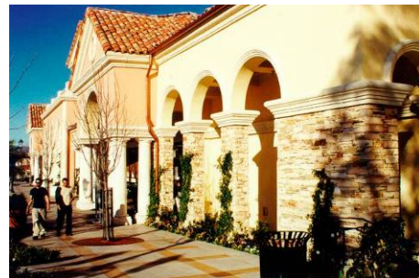
Figure 102. Articulation along wall plane.
