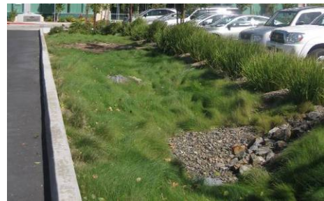
Figure 50. On-site storm water capture.
