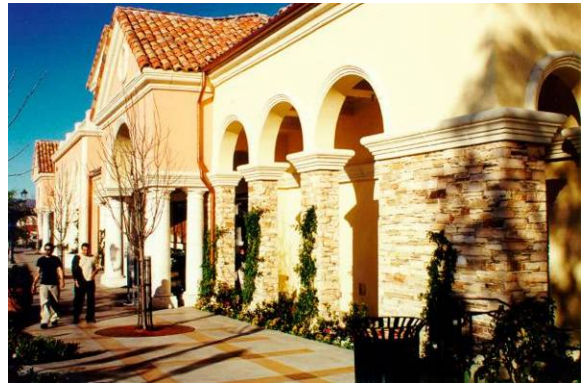
Figure 103. Articulation along wall plane.
