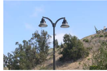
Figure 12. Hooded light fixture directs light downward.
