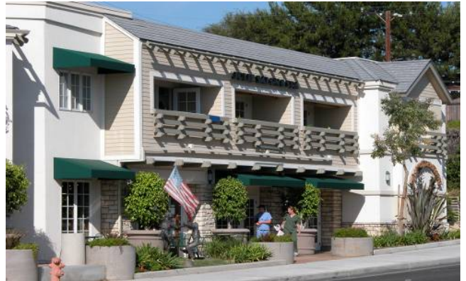
Figure 57. Building elements add visual interest.
