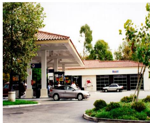
Figure 98. Sloped roof on pump island canopies.
