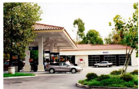
Figure 98. Sloped roof on pump island canopies.
