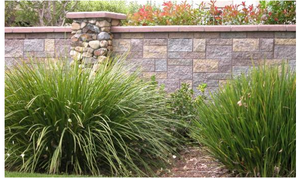
Figure 40. Wall incorporates pilasters and cap.
