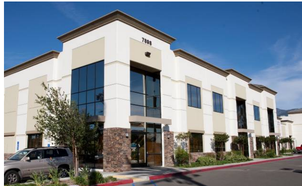
Figure 83. Awnings articulate entries to tenant spaces.
