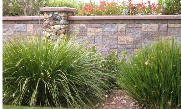
Figure 40. Wall incorporates pilasters and cap.
