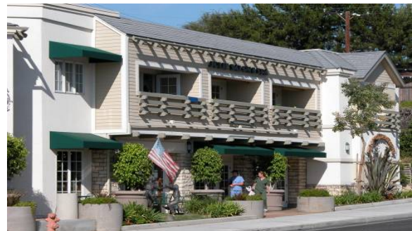
Figure 57. Building elements add visual interest.
