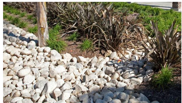
Figure 79. On-site stormwater capture system.
