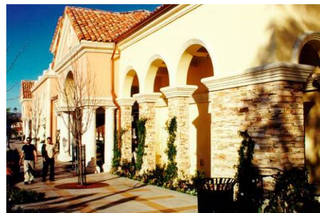
Figure 103. Articulation along wall plane.
