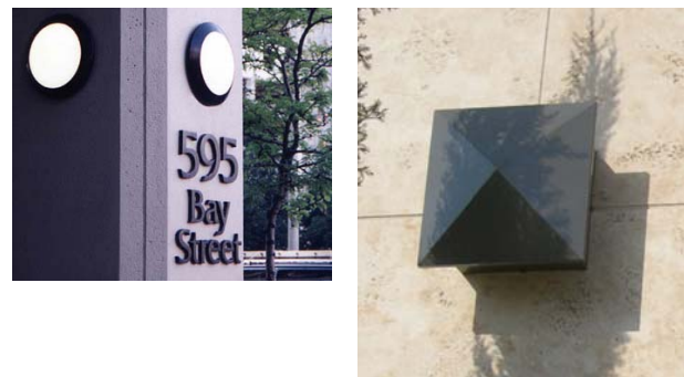
Figure 14. Decorative light fixtures.
