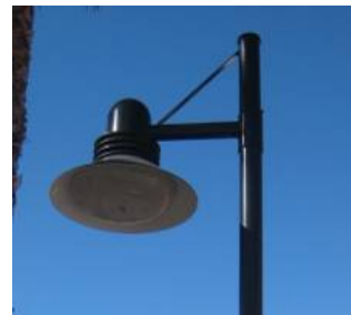
Figure 46. Pole mounted light.
